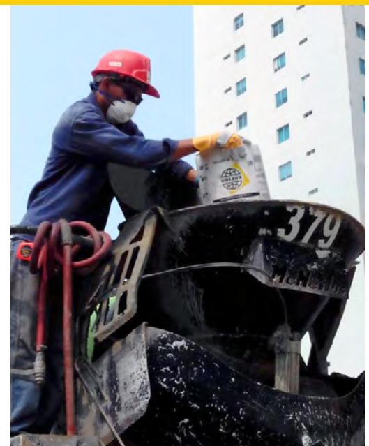
KIM is added to the concrete before placement
