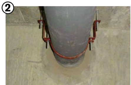
2 Waterproof pipe penetrations and tie-holes with Krystol Waterstop Grout™.
