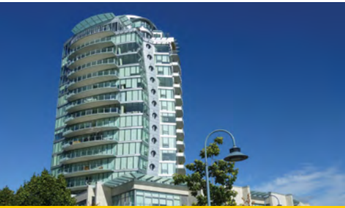
The Erickson Underground Parking Vancouver, B.C., Canada
