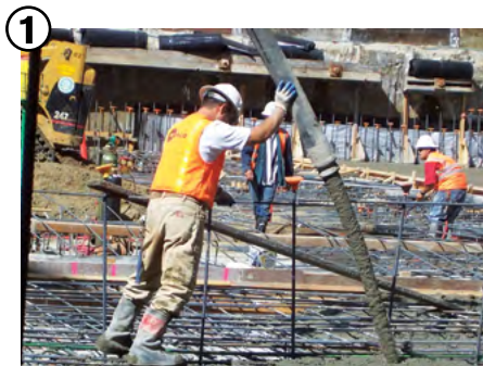
1 Create a watertight structure by using Krystol Internal Membrane™ (KIM®) in precast, cast-in-place or shotcrete walls and slabs. KIM builds the waterproofing right in to the concrete, eliminating the need for unreliable membranes.
