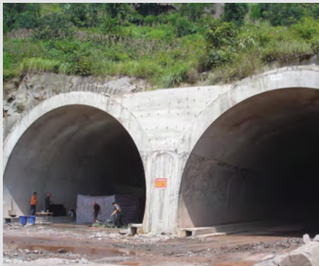
Repair work on the Yunnan Shuima Tunnels
